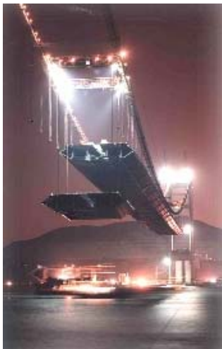
Figure 1. A section of Tsing Ma Bridge being lifted, before joining.
